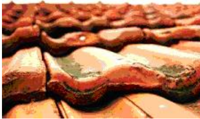
Asbestos cement roofing shingles
